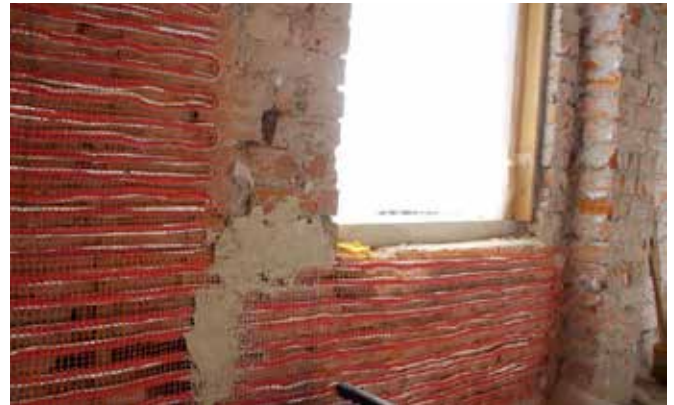
HEATER APPLICATION ON A BRICK WALL
