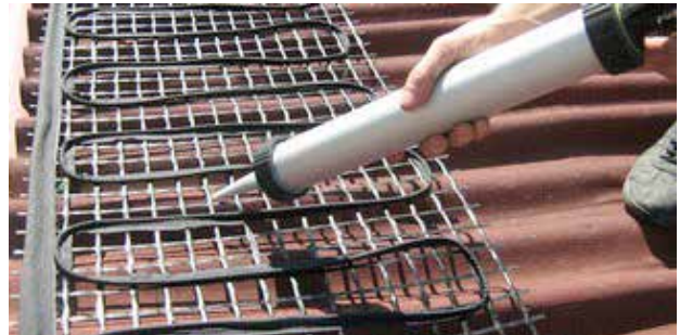
FIXING ON THE ROOF BY MEANS OF SPECIAL SILICONE
