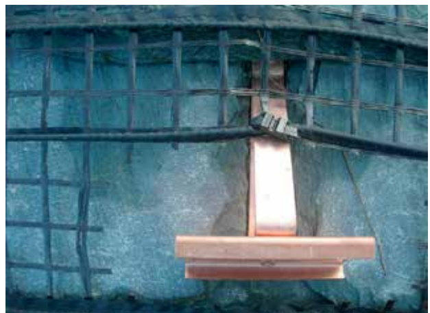
HOOKING USING A ZIP TIE ON A SNOW BARRIER
