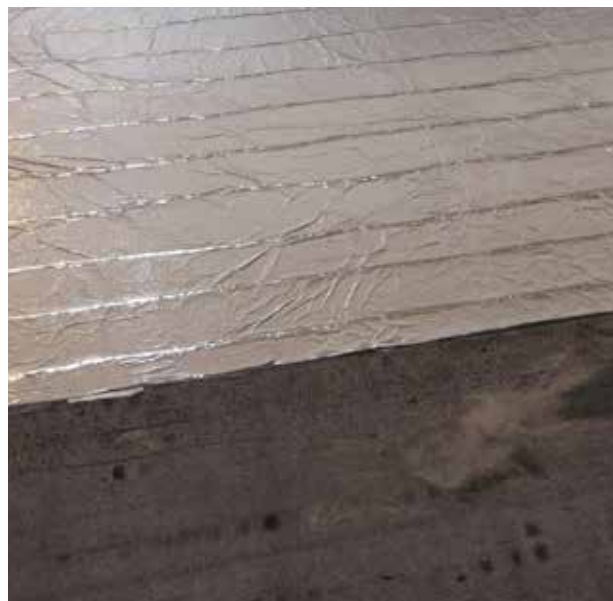
SNOW MELTING SHEET INSTALLATION
