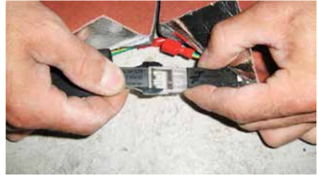
MODULE CONNECTION USING IP67 CONNECTORS
