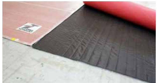
HEATING ELEMENTS LAID OVER THERMAL INSULATION SUPPLIED
