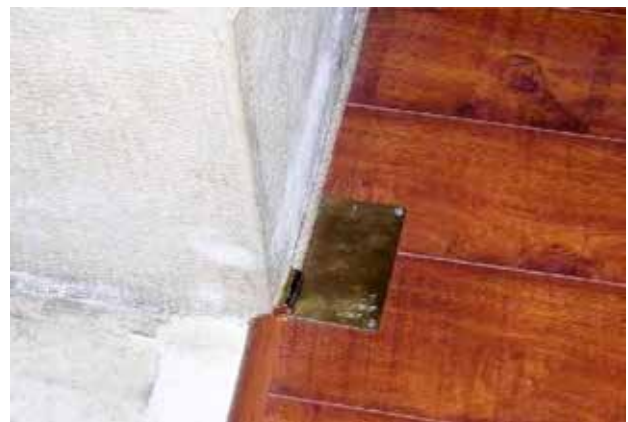
HOUSING AND COVER OF THE DERIVATION BOX MADE OF BRASS
