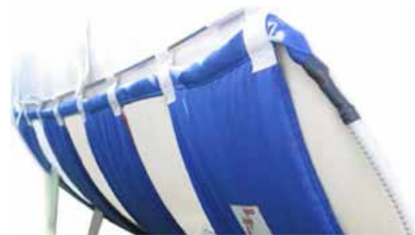
HEATING BLANKET INSTALLED ON A TANK
