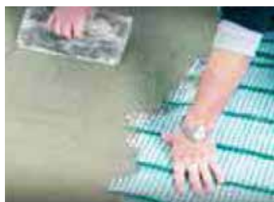
MESH LIGHT COATING FOR FIXATION
