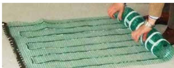
UNROLLING THE MESH ON THE PAVEMENT
