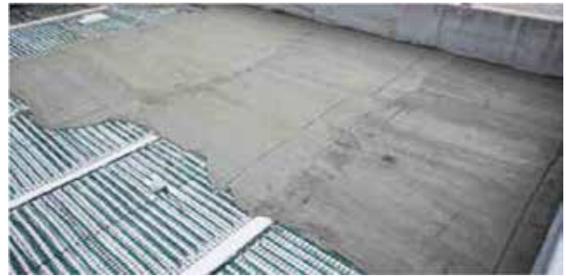
RECOATING SNOW MELTING MESH
