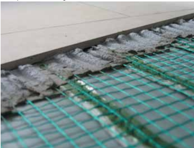
Examples for heating mesh installation
