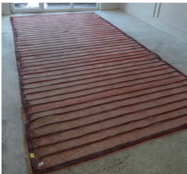
HEATING MESH LAYED ON THE FLOOR
