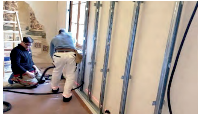
INSTALLING METAL FRAMES
