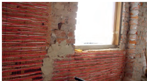
HEATER APPLICATION ON A BRICK WALL
