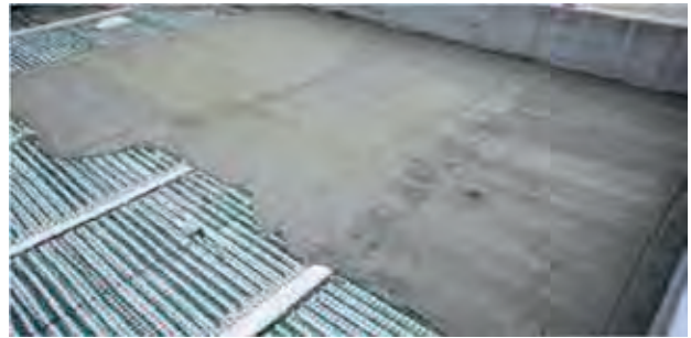
COVERING SNOW MELTING MESH
