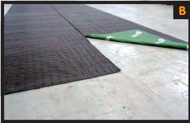
B. At the beginning lay down the elements for thermal insulation and floor protection, make sure the installation surface is flat and clean. The elements must be laid side by side, they must not overlap and/or fold upon each other, the elements must not be larger than the surface to be heated.
