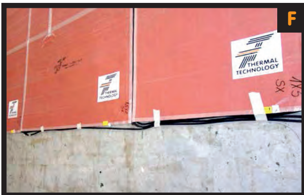
F. Pass the cords under the element's boards, or between two elements, where possible.
