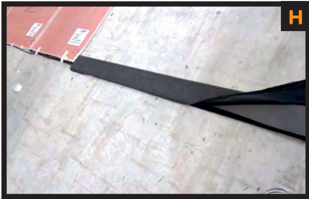
H. Close the duct using the lid and wrap it using the elastic and anti-slippery material, both provided.
