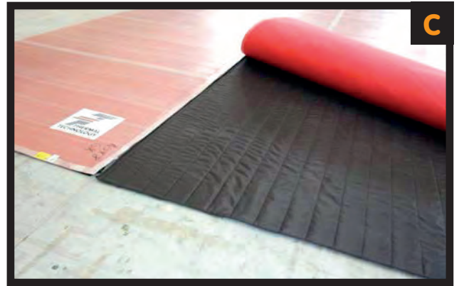
C. Place the heating elements over the thermal insulation.
