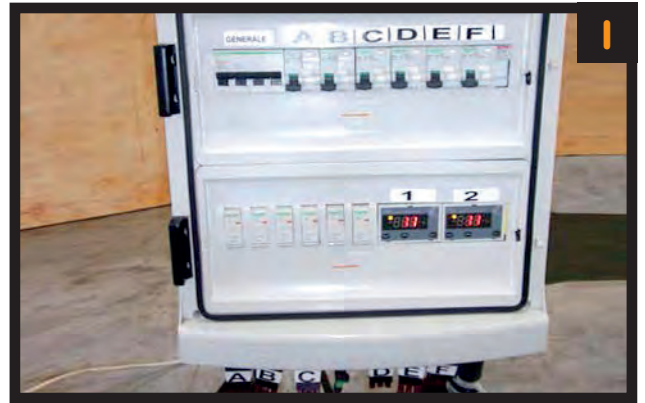
I. Connect the power cords and probe cords to the appropriate circuits on the electric board
