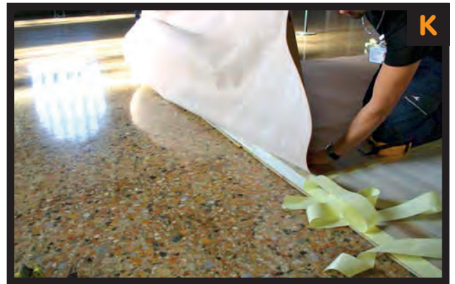
K. Once verified the functioning of all the elements, place the moquettes using common bi adhesive band.
