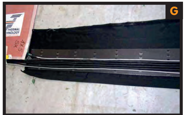
G. The cables must be grouped in the point indicated on the project, and an appropriate protection duct must cover them until electric board.
